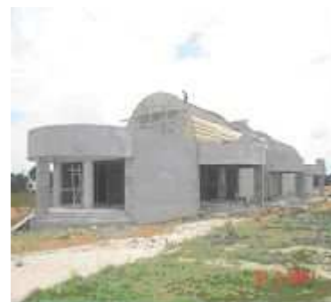
The facility is set to be finished in late 2006
